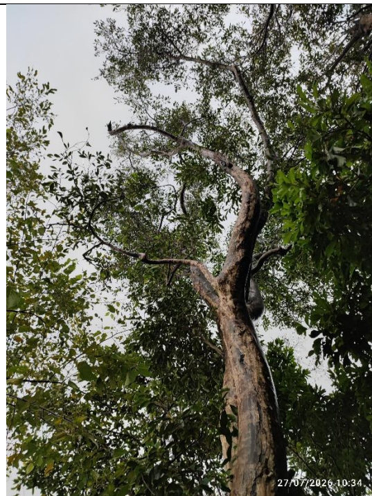
U041 – Crown condition
