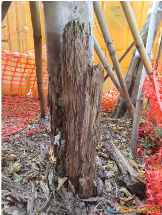
11: U041_Wood damage at trunk union#2
