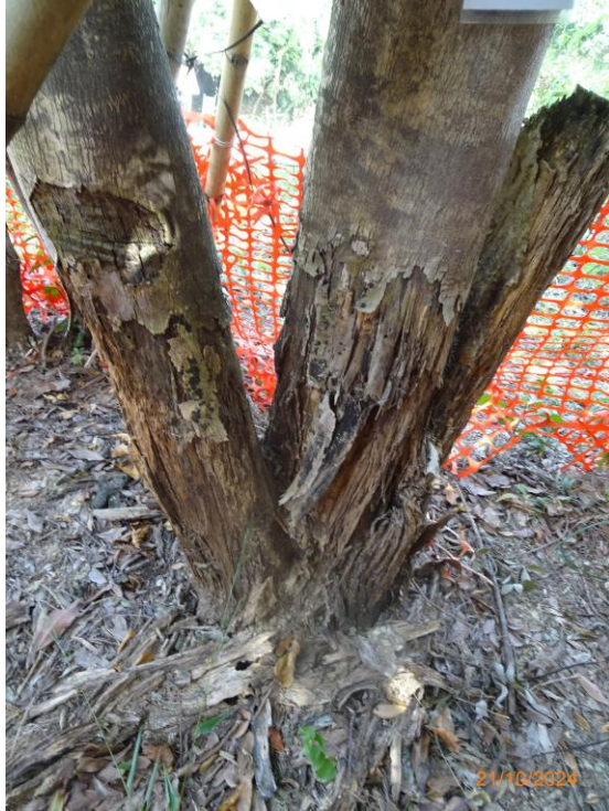
13: U041_Wood damage at trunk union#3
