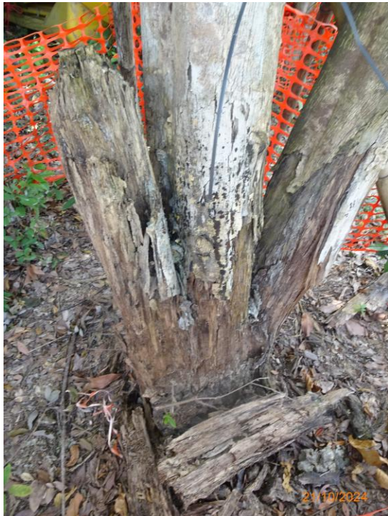
11: U041_Wood damage at trunk union#1
