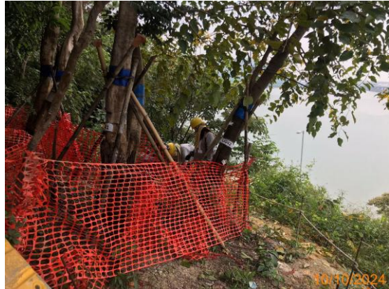
26: Temporary protective fencing for U041, U042 and U043
