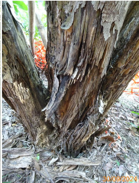
12: U041_Wood damage at trunk union#1
