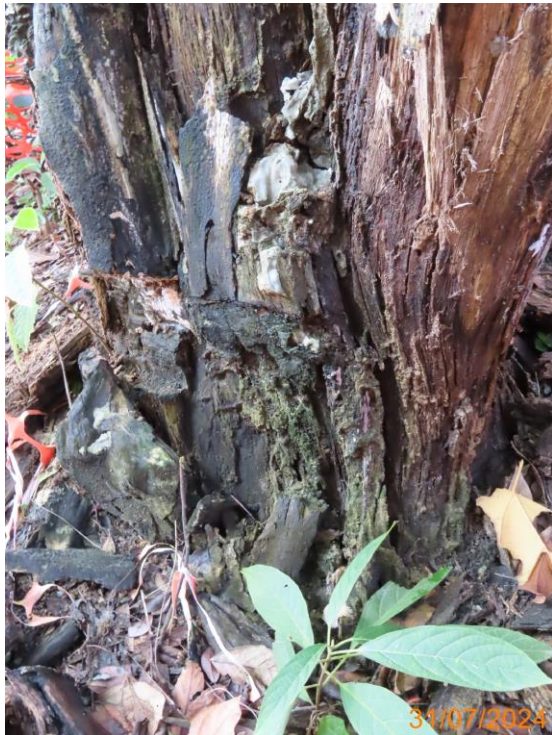
11: U041_Wood damage at trunk union
