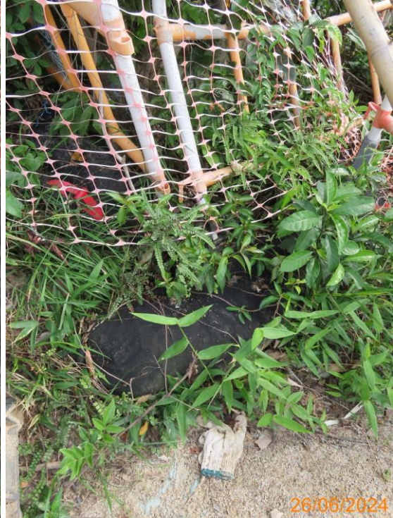
22: Slit rock and protection zone
