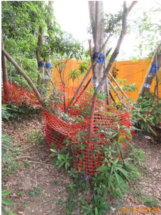
23: Temporary protective fencing for U041, U042 and U043
