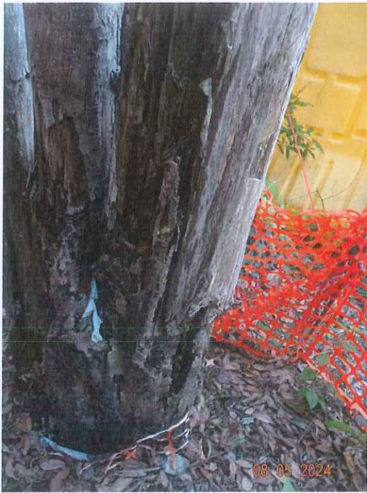
9: U041_Dead stump_Close up, crack enlarged since late March 2024, extra staking was provided on 21 March 2024
