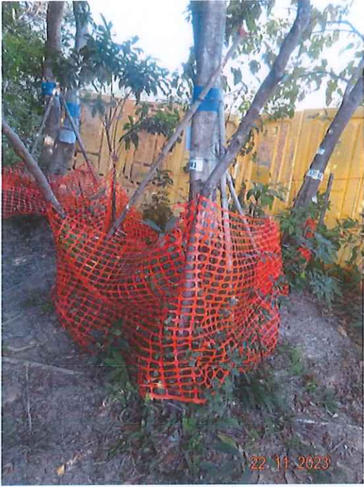
18: Temporary protective fencing for U041, U042 and U043
