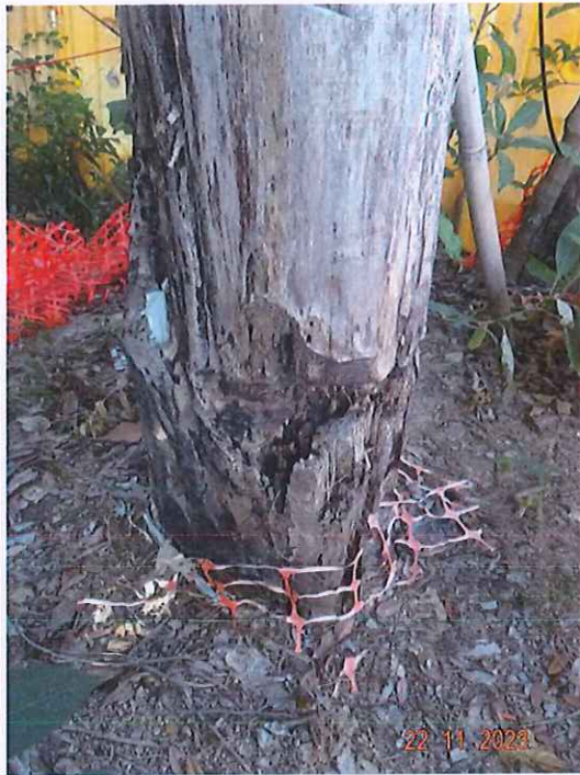
8: U041_Wood damaged by termite
