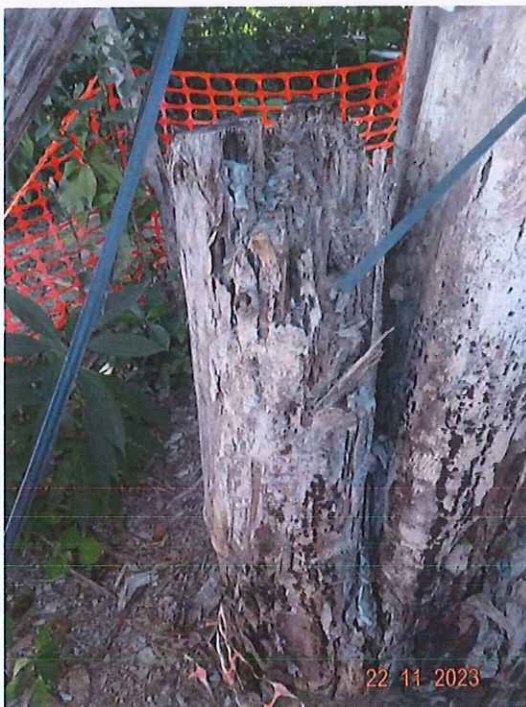
7: U041_Wood damage at trunk union
