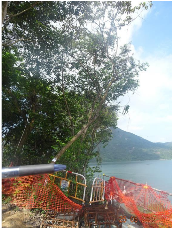
19: Protective fence which silt rock composed of woo chip is required
