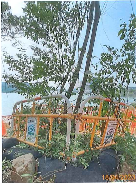
9: Protective fence sealed by silt rock composed of wood chip
