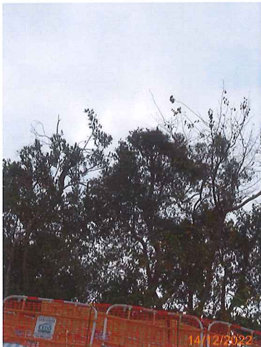
7: Temporary protective fencing for U041, U042 and U043 (2)
