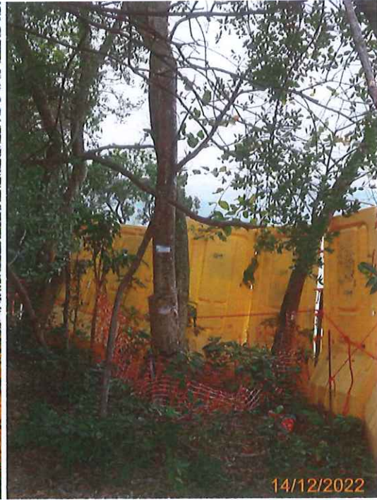
6: Temporary protective fencing for U041, U042 and U043 (1)
